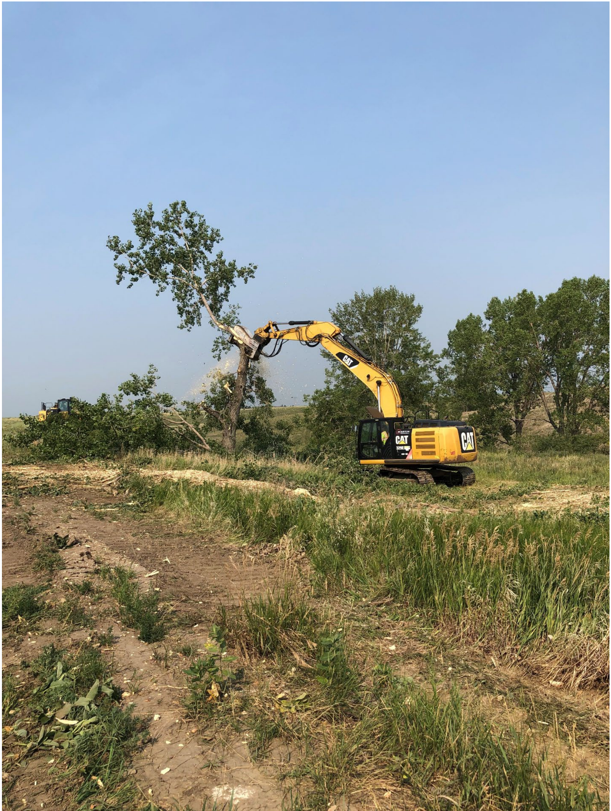
Figure 7: Trees being shredded at the Lindahl Site.
