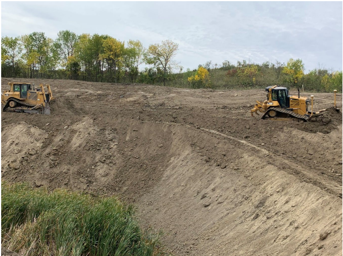
Figure 3: Dozers Moving Spoil Material at the Knorr Site.
